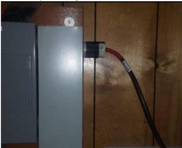
3. Unplug the 3 AC cords identified by red tape on east wall, ground level.
