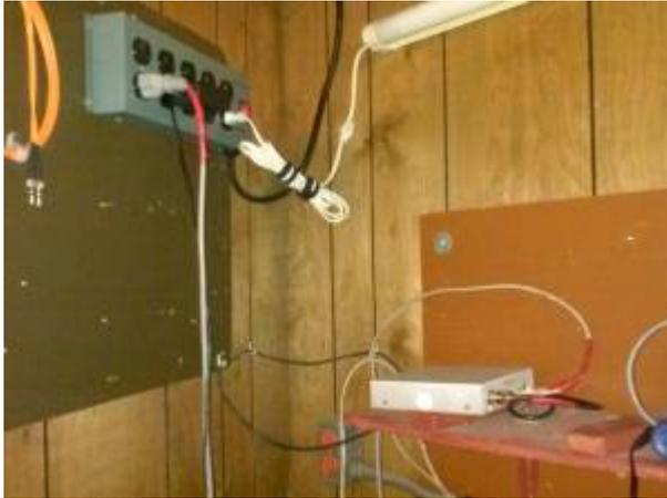
2. Unplug the one (1) twist lock plug for the laser printer identified by red tape from the sockets mounted on the west wall, chest height. Twist each connector counterclockwise towards you and then pull straight out of the socket.
