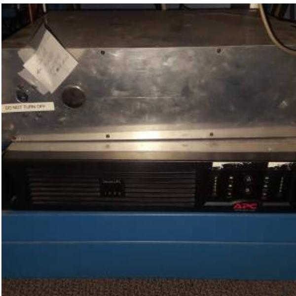
17. Unplug the UPS unit from the orange outlet on the frame below the window sill behind the telescope control console. AC cord identified by red tape
