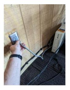
Next you must turn on the UPD. Press and hold the corresponding "on" button for at least a second until you hear a beep, then let go. the UPS will immediately supply power to their output plugs, so no further button pressing is necessary on the UPS. Last update: 2023/08/23 public:catalinas:lemmon:phillips\_24:startup\_procedure https://lavinia.as.arizona.edu/~tscopewiki/doku.php?id=public:catalinas:lemmon:phillips\_24:startup\_procedure&rev=1692819852 12:44
