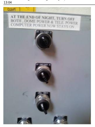
If at all possible you should stow the telescope before doing this. When this computer is restarted it will assume the Telescope is at stow
