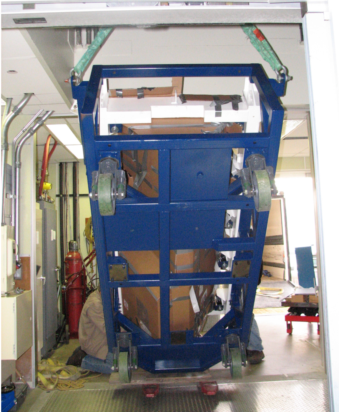
MAESTRO being lifted up through the hatch to the chamber.
